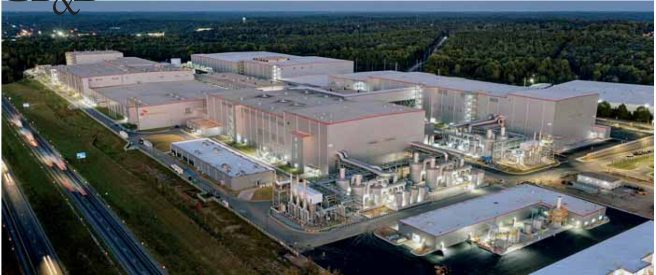
SK's EV battery plant in Jackson County, Ga., supplies batteries for a variety of automakers in the Southern Auto Corridor. It was one of the first battery plants completed in the South.
